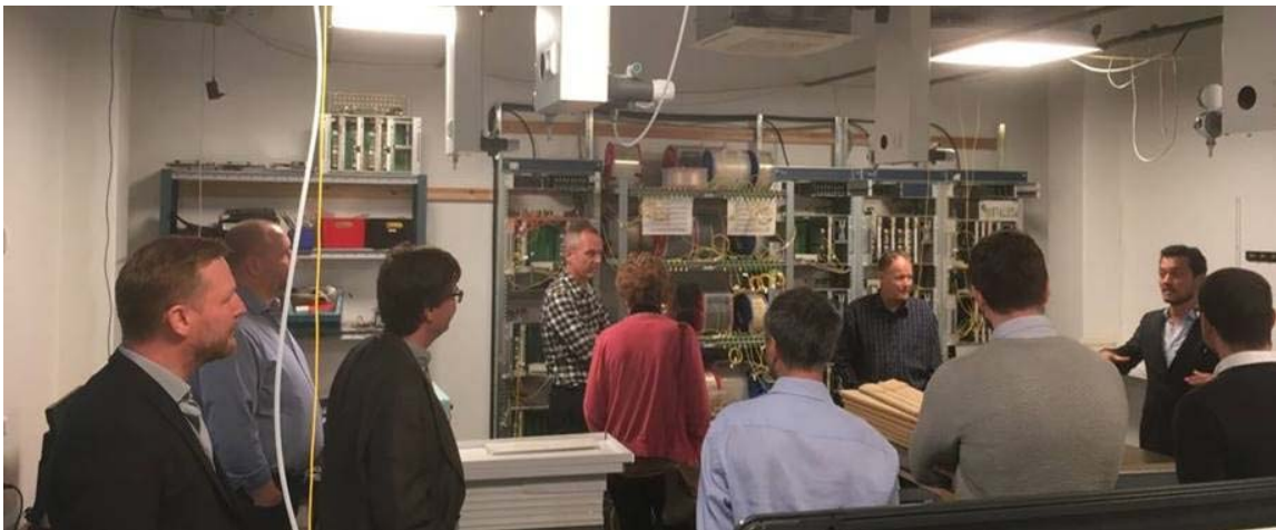
INCOM Testbed facilities at DTU Fotonik in Kgs. Lyngby (building 340)
